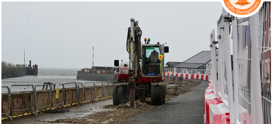
Demolishing wall at Quay Parade
