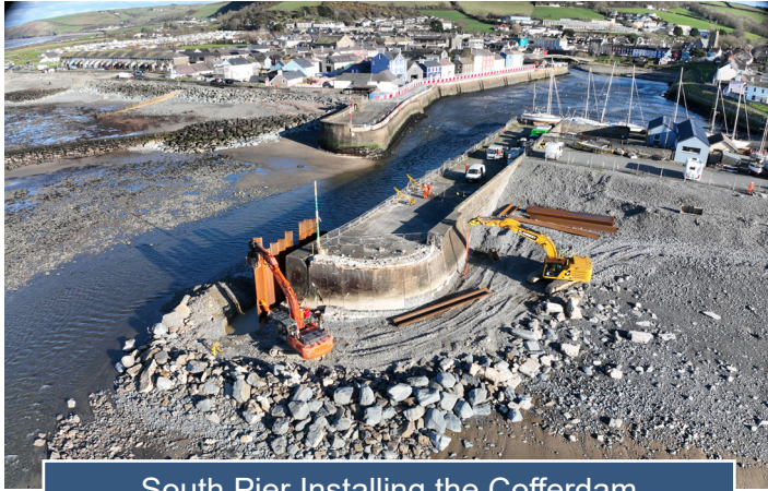
South Pier Installing the Cofferdam
