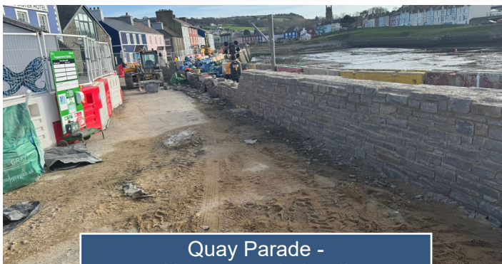
Placing the pre-cast units along the breakwater
