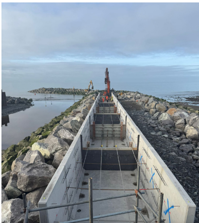
Placing the pre-cast units along the breakwater
