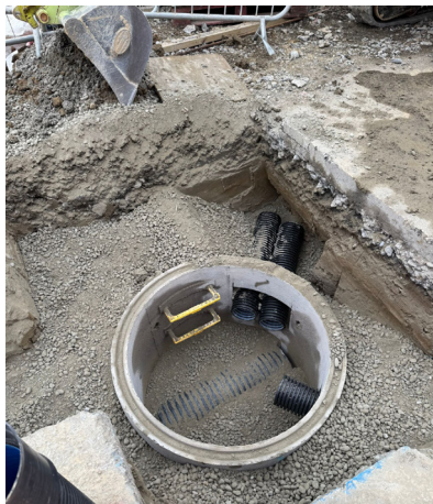
Quay Parade - Setting new drainage manholes
