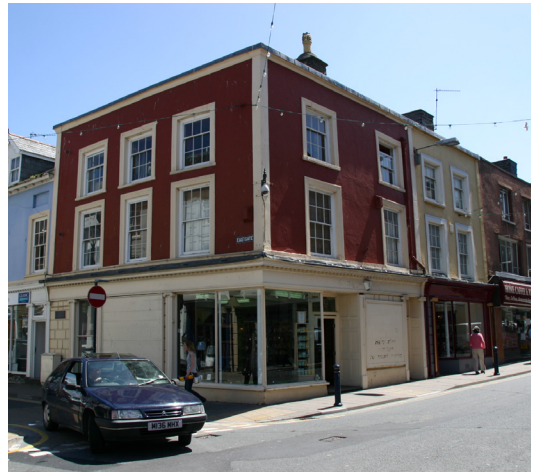
17-19 Pier Street before TIG funded building improvements.
