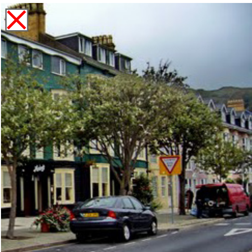
Box dormer windows do not match others in the street and are not acceptable.
