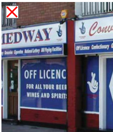
'On window' signage completely obscures views into the shop creating an oppressive and unwelcoming shopfront
