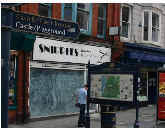
Poor quality and out of scale signage has a negative effect on the appearance of the Conservation Area
