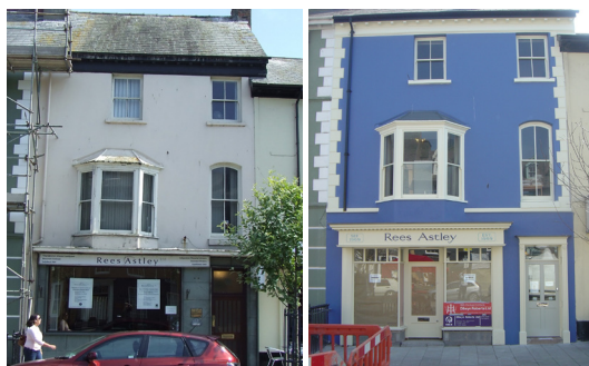
Eastgate: A simple and restrained shopfront with a domestic scale before and after restoration.
