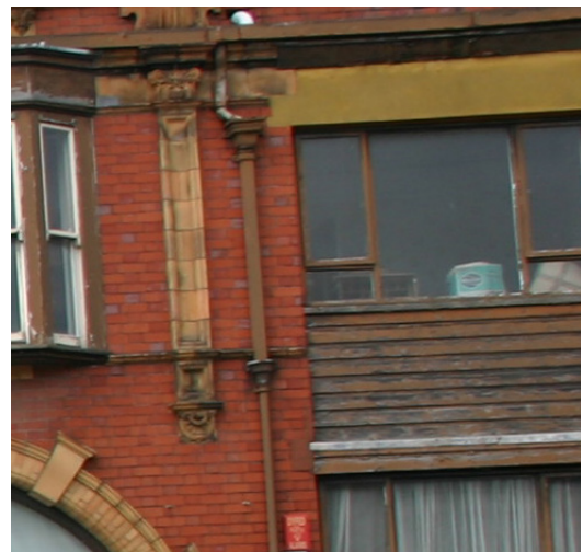
Example of an original downpipe with decorative hopper head
