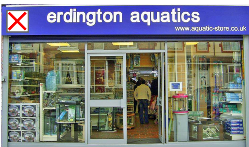
A lack of stallriser results in a poor quality shopfront and doesn't frame displays well.
