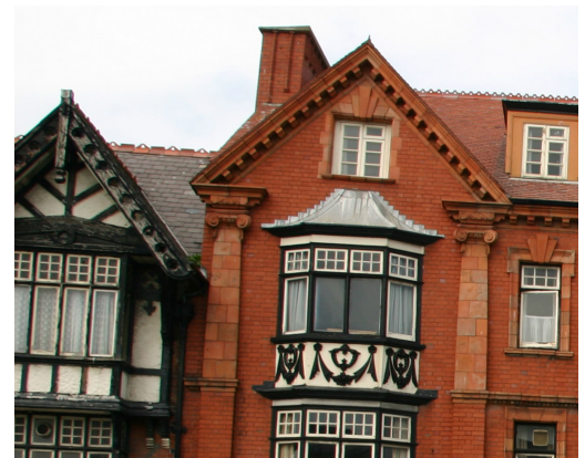
An example of a slate roof and a red clay tile building in close proximity. Both buildings have deep eaves with ornate brackets
