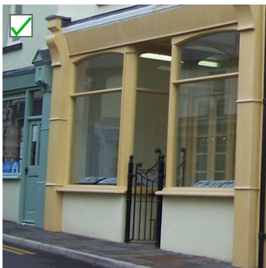
An example of the retention and refurbishment of existing decorative security gates
