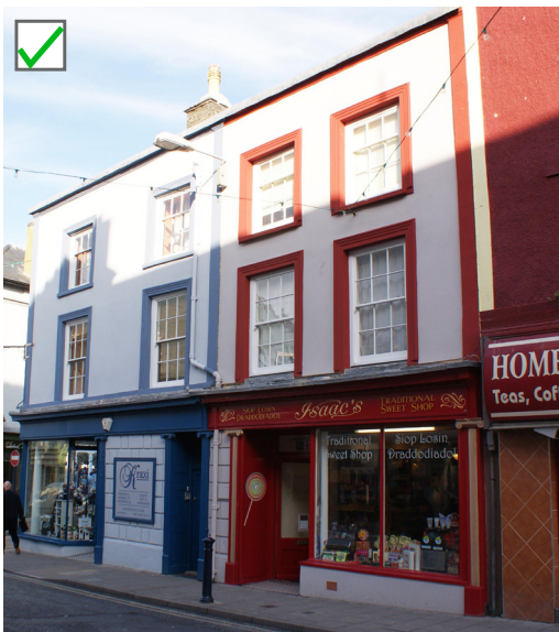
Vertical masonry bands in a continuing colour extend from the pilasters to further define and 'frame' the upper floors
