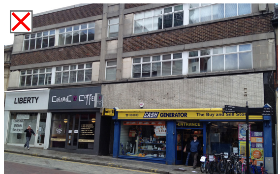
The shopfront to the right is an 'off the shelf' design and its Victorian proportions pay no regard to the proportions of the building or adjacent shopfronts
