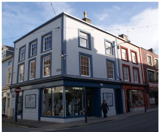
17-19 Pier Street after. Improvements are of high quality and are appropriate to the building and its surroundings
