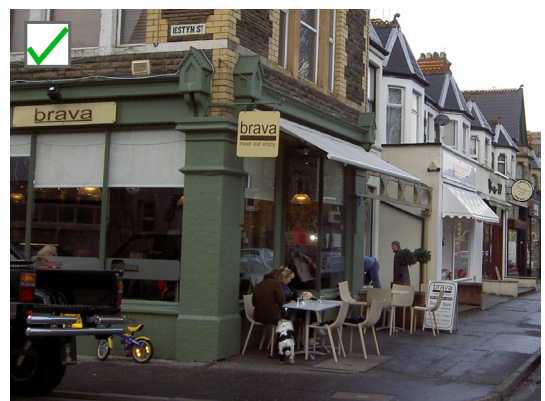
Traditional roller blinds which can be discreetly hidden away within a fascia providing an attractive and usable space in front of the retail unit
