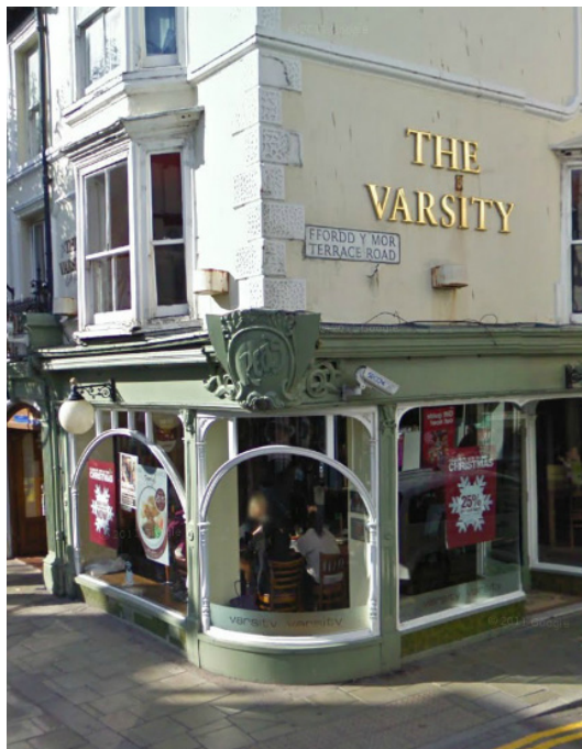
An example of a good quality and prominent corner building which retains most of its original shopfront elements.
