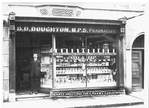
This historic photo shows a pharmacist in Aberystwyth which adopted a low stallriser to display their goods
