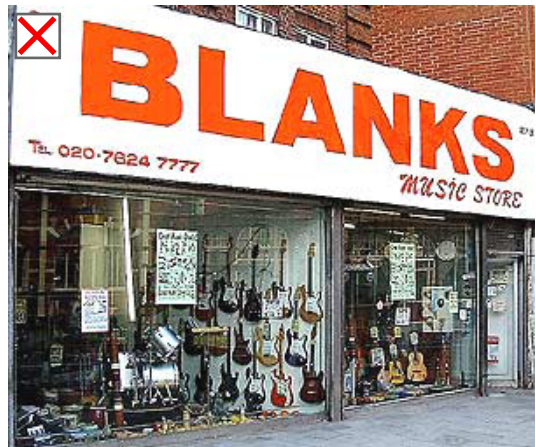
This poor quality fascia dominates the shopfront
