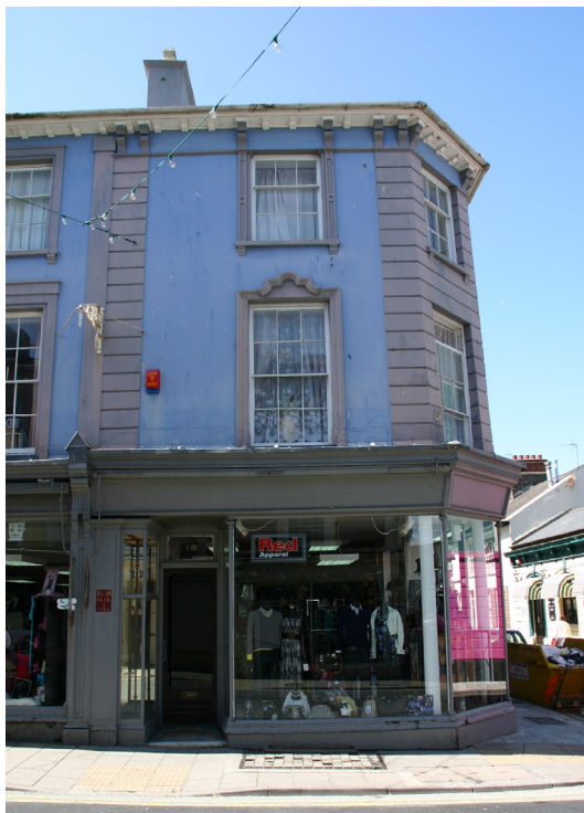
An example of a traditional shopfront in the heart of one of the original commercial areas on Pier Street.
