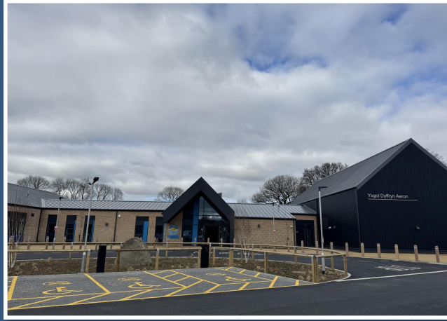
The new Ysgol Dyffryn Aeron was officially opened in March 2025 providing modern, state of the art learning facilities for pupils
