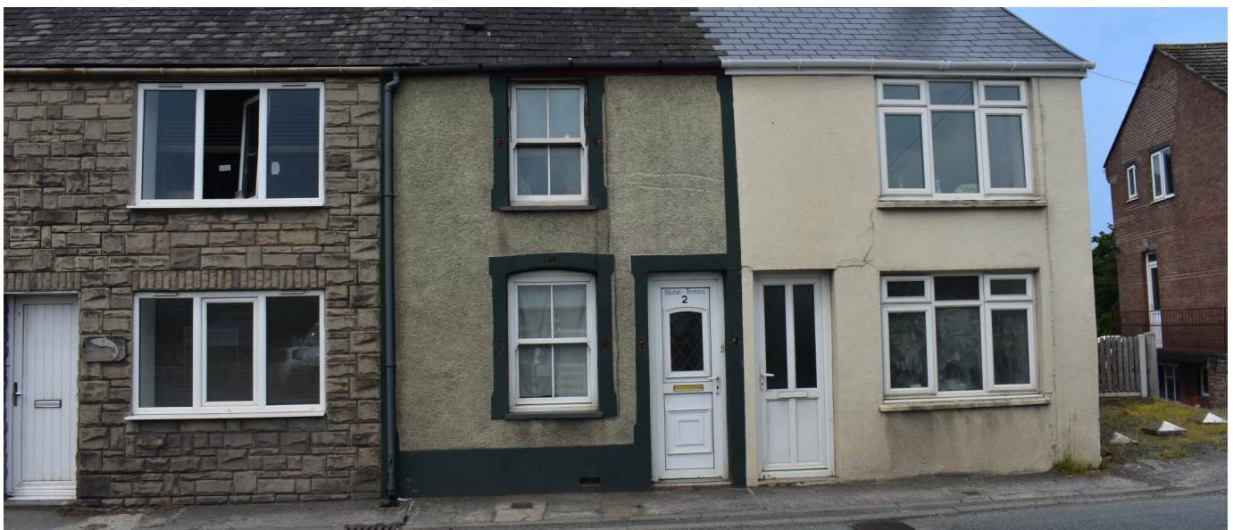
Fig. 37 The loss of traditional windows and doors, cladding and cement render negatively affects the character and appearance of traditional cottages
