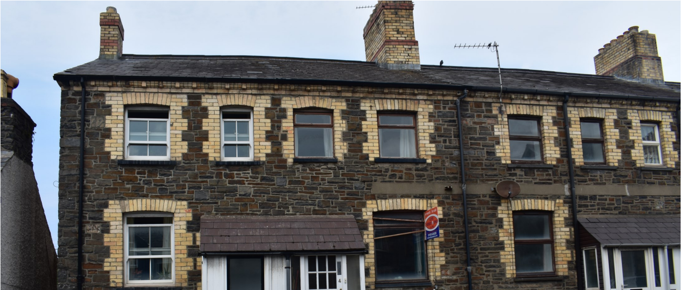
Fig. 25 Contrasting brick details around windows and doorways and chimneys add distinctiveness to separate rows of terraces
