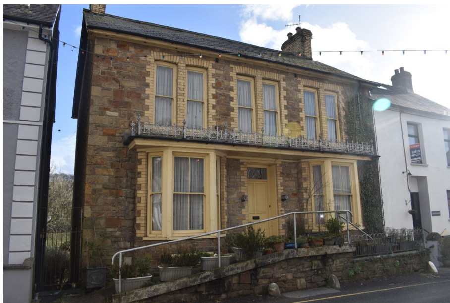
Figs. 37 & 38 Two houses of the same period - adjoining - one with original windows, door, ironwork and stone boundary wall incorporated into improved disabled access. The other with modern Upvc windows, door, concrete render, rooflight, altered door and window openings and lost front boundary wall.
