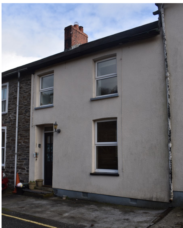
Fig. 35 Traditional cottage with new windows, door, concrete render, fibre roof tiles, concrete steps
