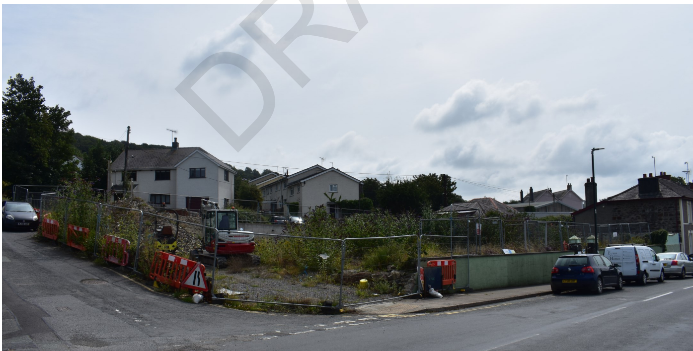
Fig. 5 Design guidance is needed for potential development sites both within and in the setting of the conservation area
