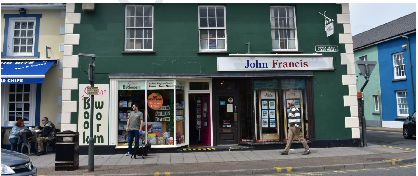
Fig. 6 Historic shopfronts positively contribute to the character of the area but some modern signage negatively impacts on these positive features
