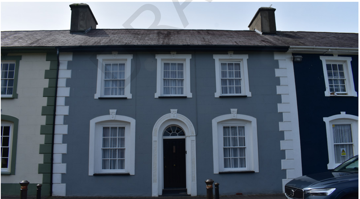
Fig. 16 Traditional Georgian style classical features: equal proportions and regularly and symmetrically placed features, small pane sliding sash windows, architrave with key stones around windows and door, quoins, classical references in the doorcase, arched fanlight above the door, six panel solid door set above pavement level with steps, low deep ridge chimneys at the end of each terrace, low pitched natural slate roof.
