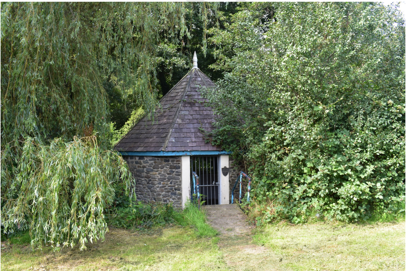
Fig. 4 The Chalybeate Well Building
