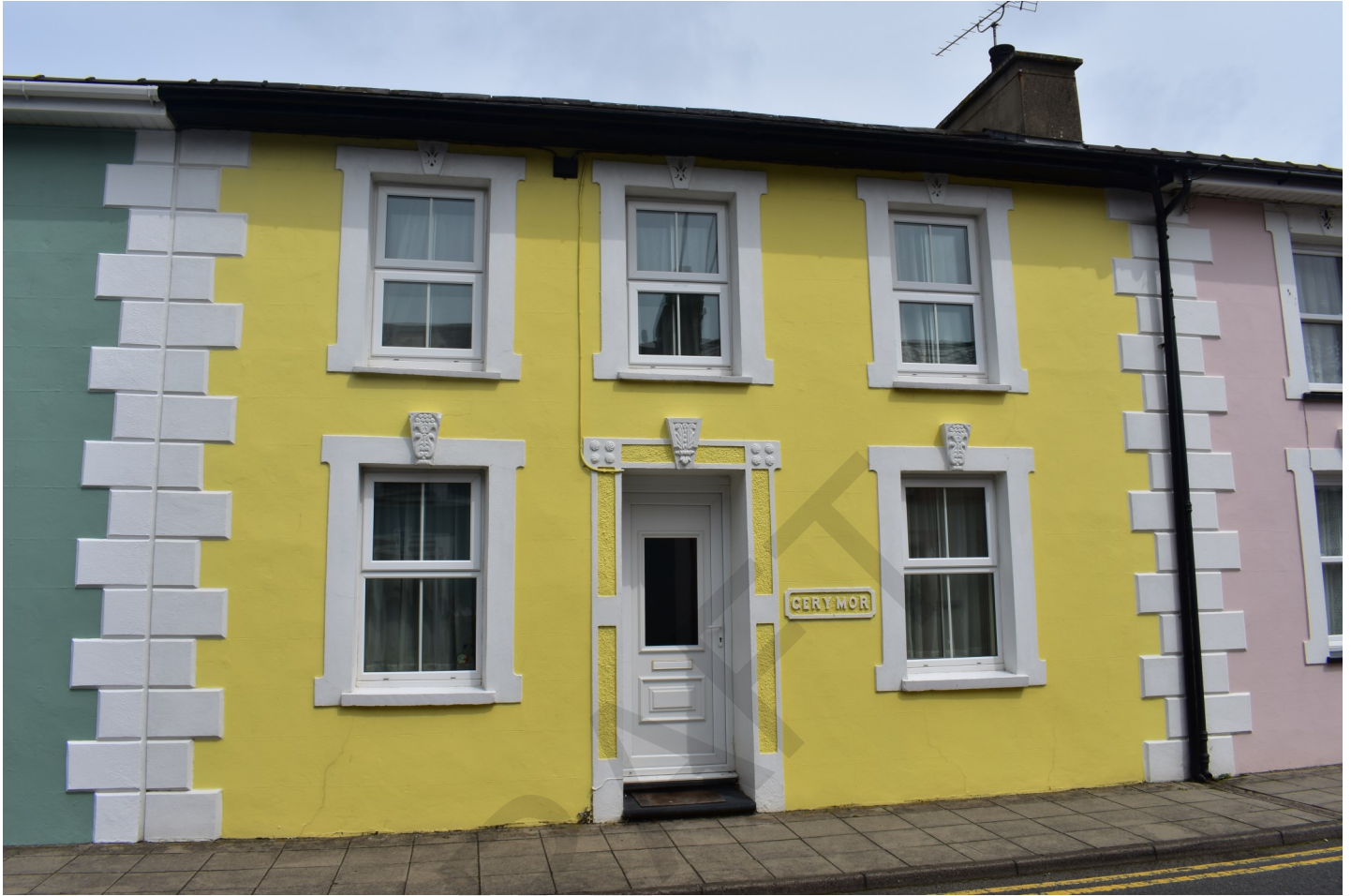
Fig. 2 Inappropriate replacements of traditional features such as windows and doors can negatively impact on the individual building and the character and appearance of the wider conservation area
