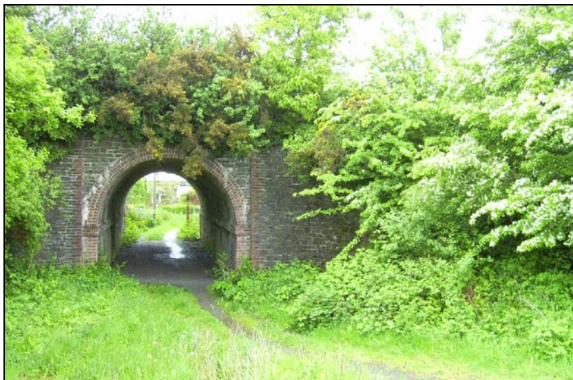
Figure 4.3 – One of Underpasses through Railway Embankment
