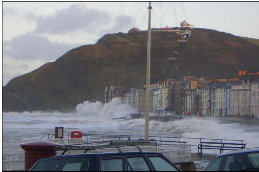
Figure 4.2 - Wave Overtopping at Victoria Terrace (January 2005)
