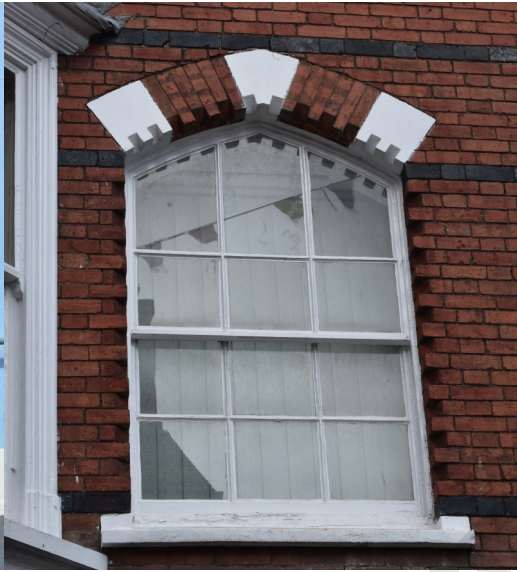
Fig. 19. Georgian style sash in Victorian gothic façade
