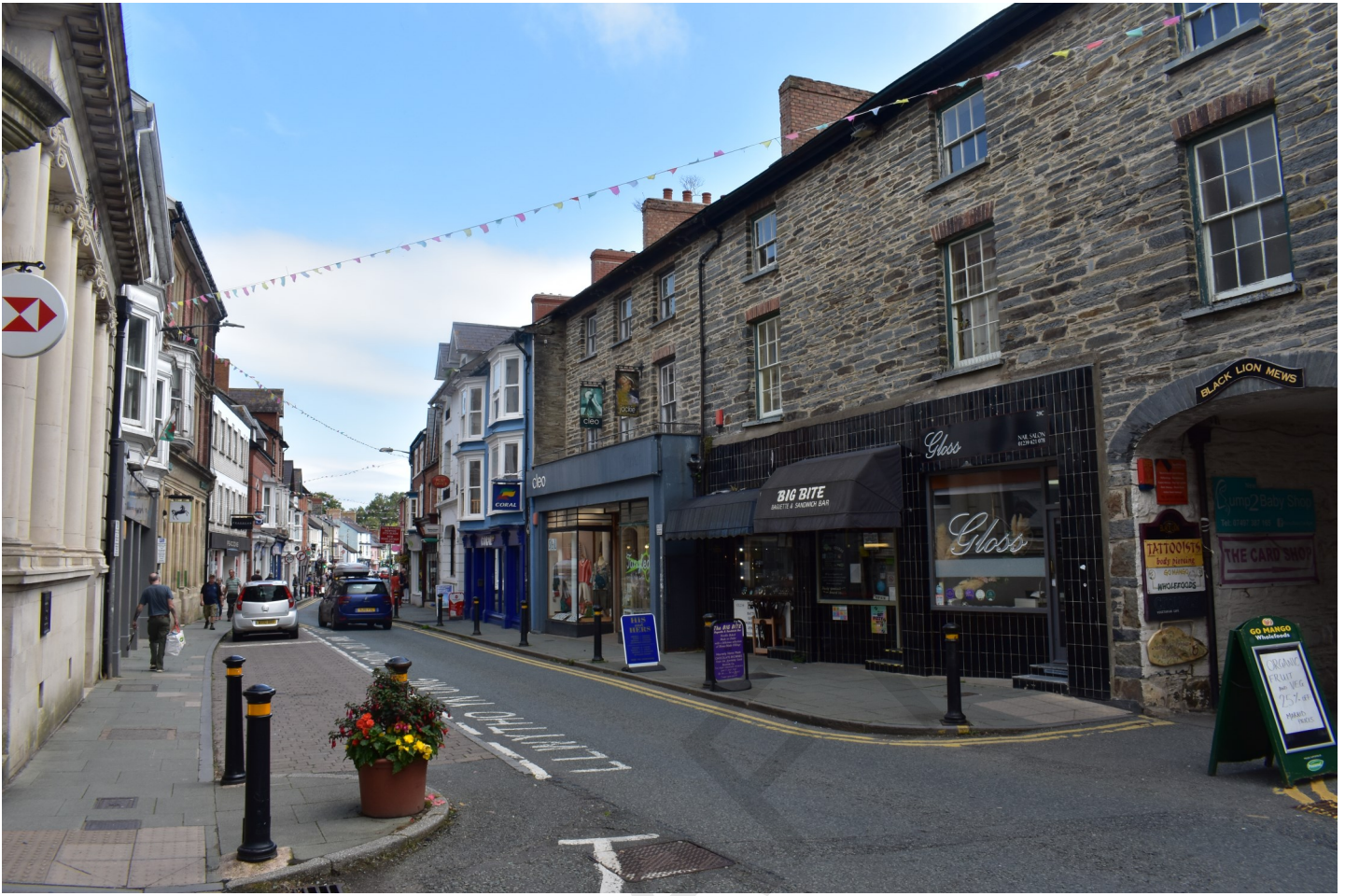
Fig. 16 It is important to build on previous successes and work in partnership with other stakeholders to ensure the historic town centre remains attractive, vibrant and sustainable
