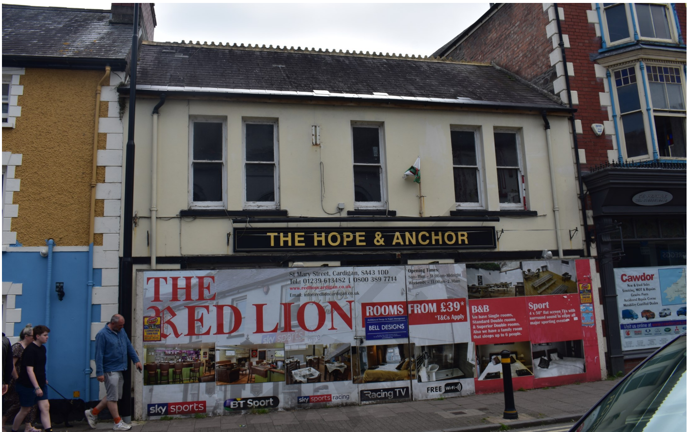
Fig. 7 Despite their historic significance, empty buildings can detract from the aesthetic value of the conservation area
