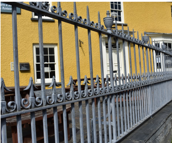
Fig. 27 Historic iron railings
