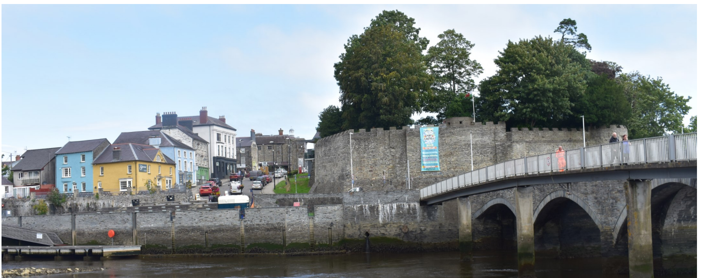
Fig. 2 View of part of Cardigan Conservation Area across the Teifi
