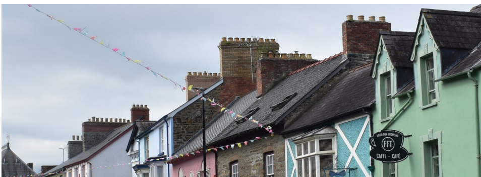
Fig. 26 Large chimney stacks punctuate the skyline
