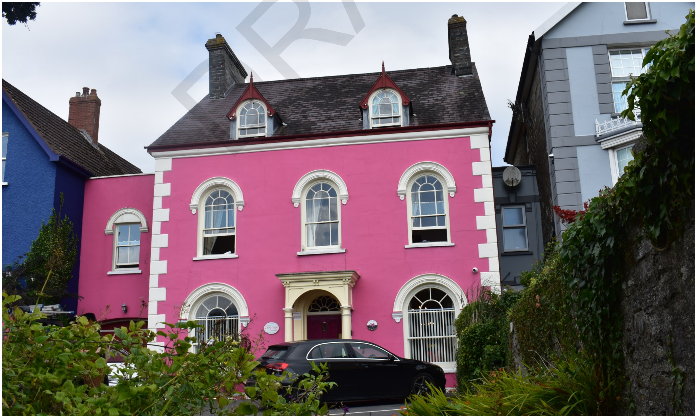
Fig. 8 There are many sympathetic ways in which traditional buildings can be upgraded to improve their thermal performance without damaging significant features
