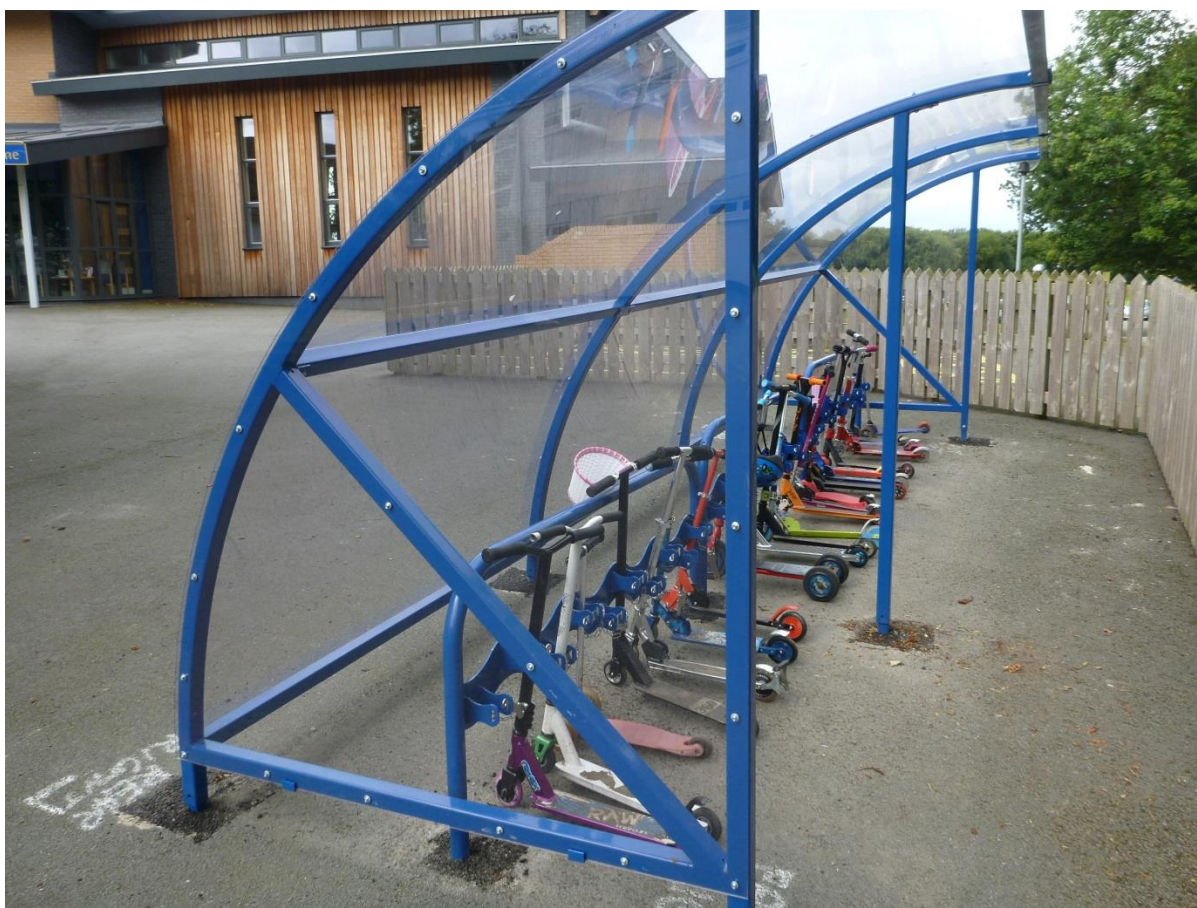
Below: New scooter shelter installed at Plascrug Primary School.
