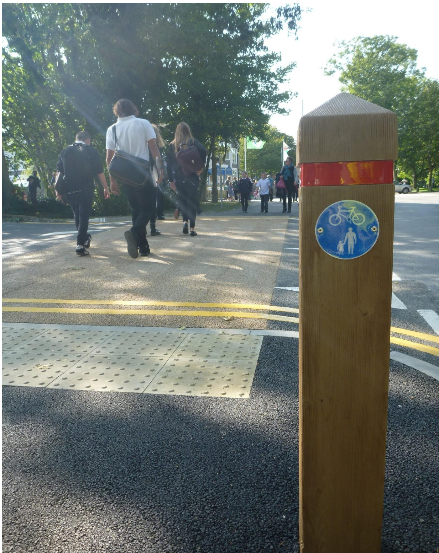
Below: New raised table crossing at entrance to the Rugby Club near Plascrug Primary School.
