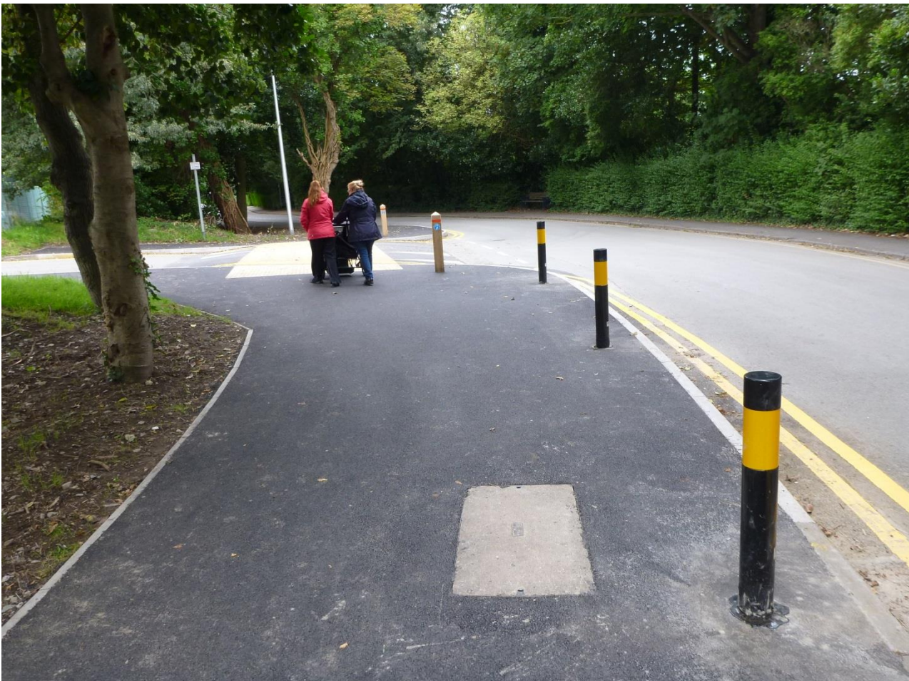
Above: Pre-scheme. Below: New raised table crossing with reduced width crossing distance and tighter junction radii. New bollards and wider shared use path with new tarmac surface.
